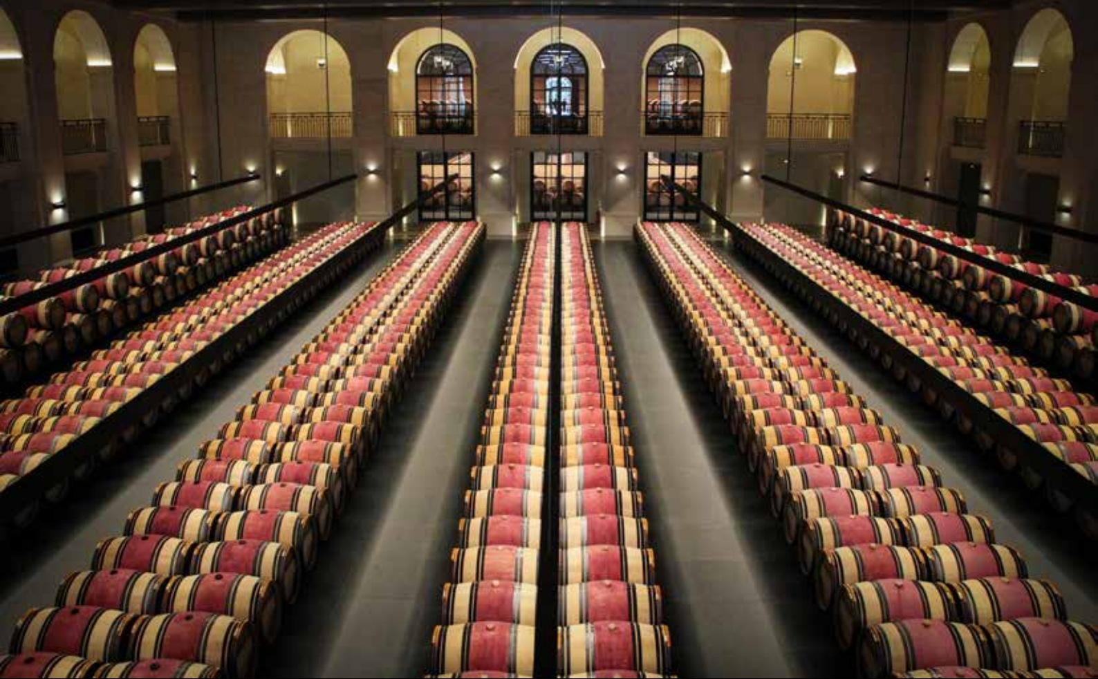
New cellar at Chateau Montrose
